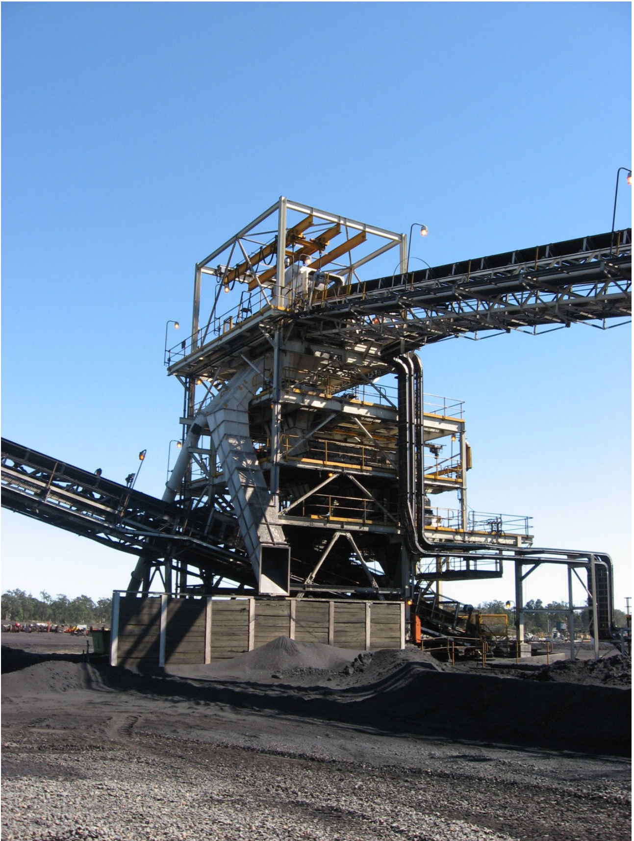
Plate 5. Typical Crusher / Sizer
