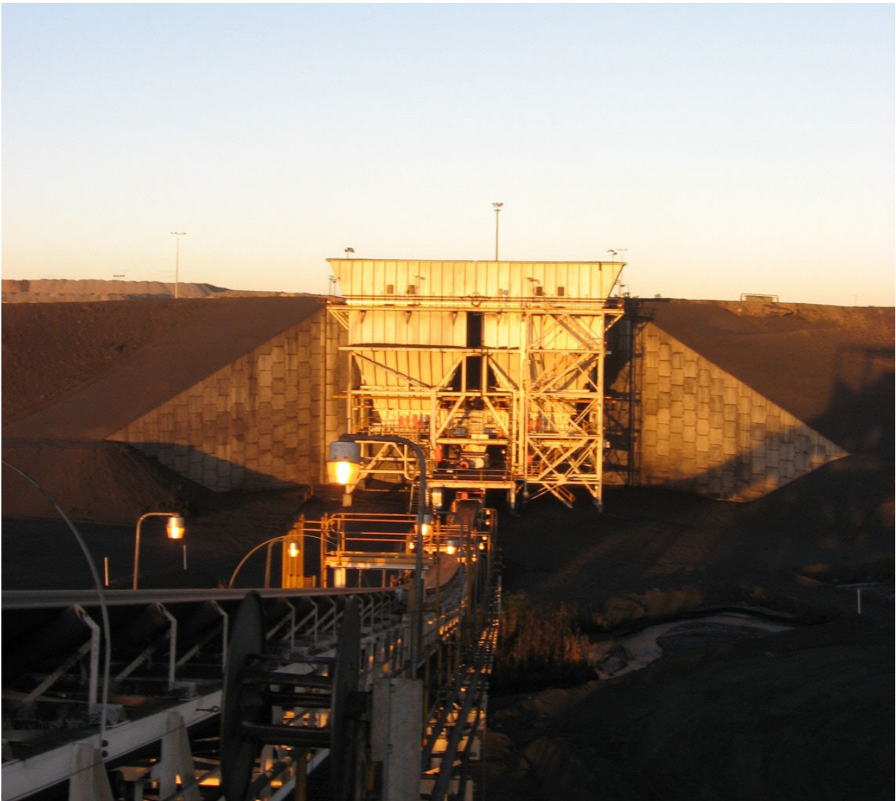
Plate 4. Typical Open Cut ROM Dump Station
