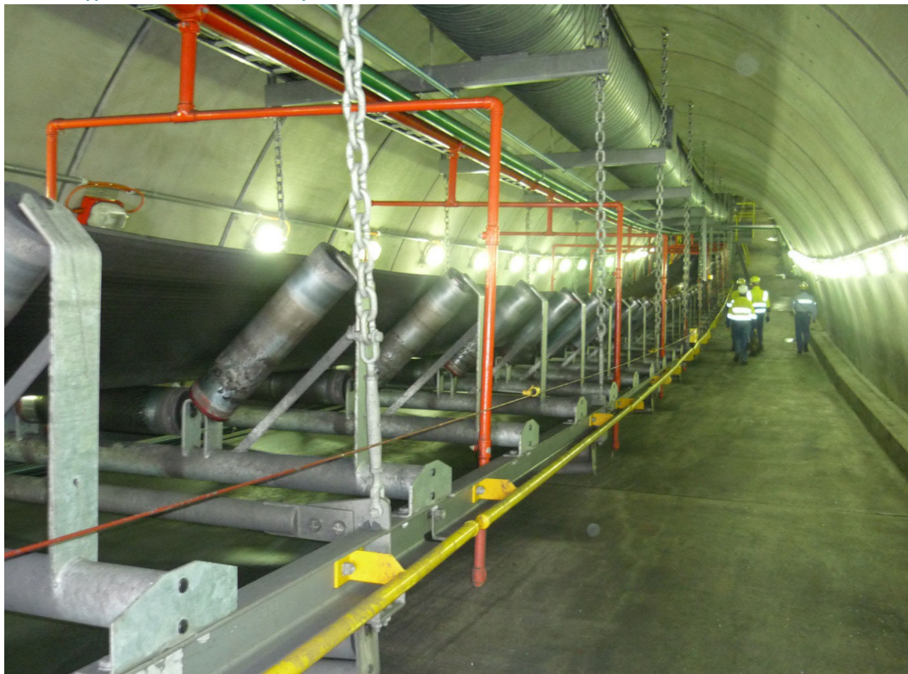
Plate 6. Typical Trunk or Drift Conveyor
