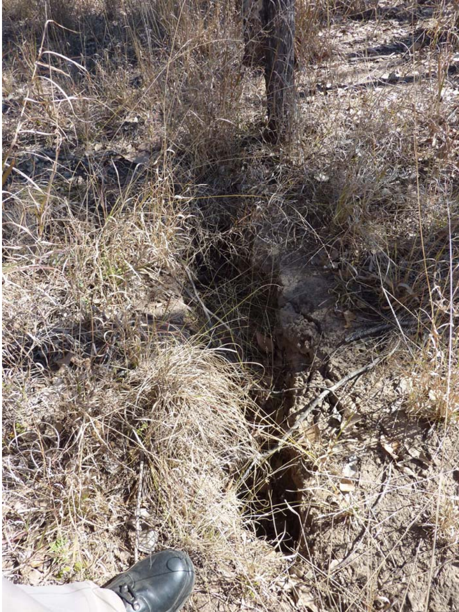
Fig. 5.6 Typical crack along longwall commencing at approx. 300m cover
