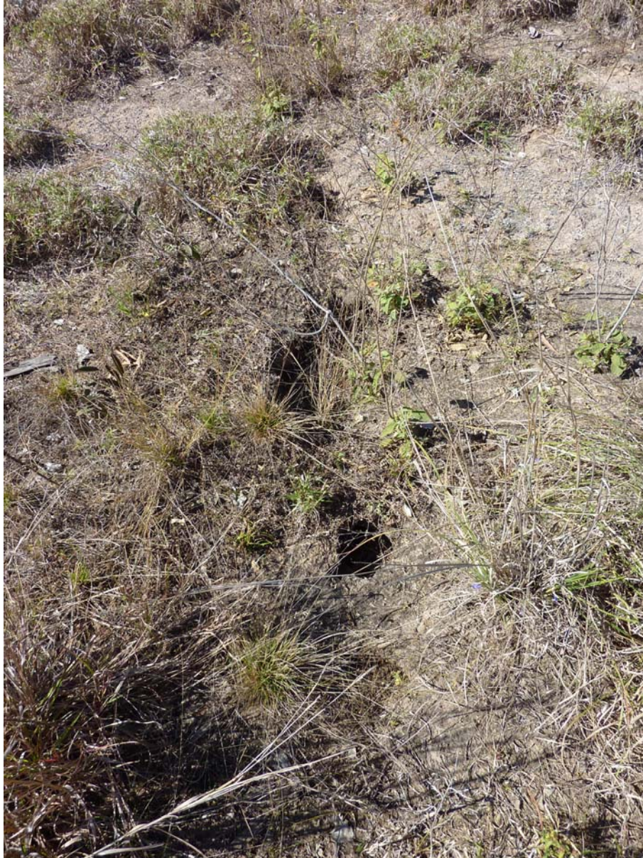
Fig. 5.7 Typical crack along Longwall commencing end at approx. 300m cover
