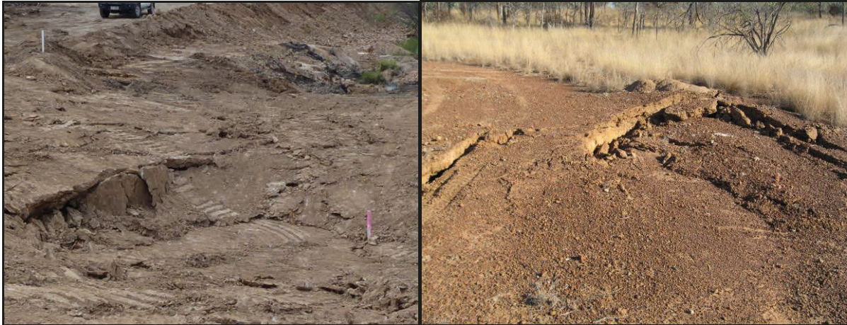
Figure 40. Heaving and Buckling.
