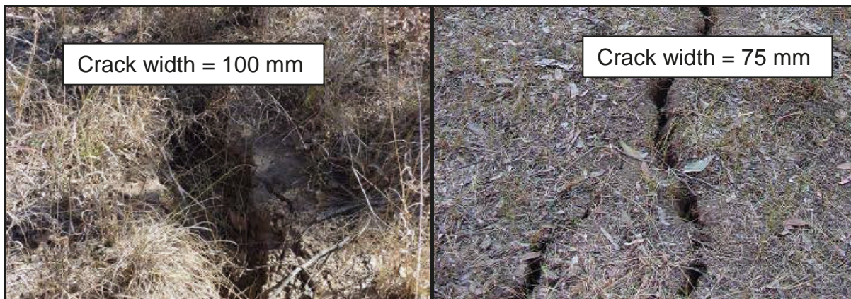
Figure 39. Examples of Subsidence Cracks.
