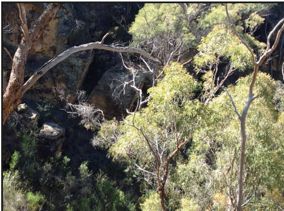
Figure 49. Failure of Clematis Sandstone along a Joint Plane.
