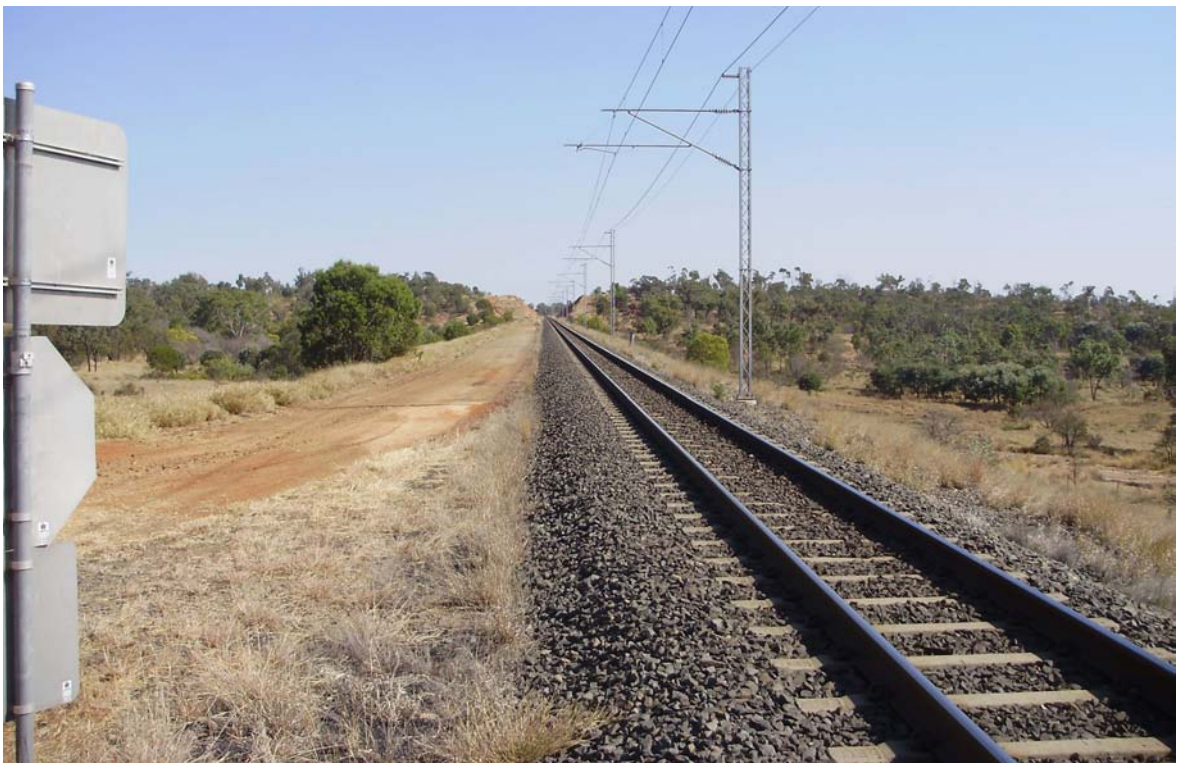
FIGURE 6 Wilton Project area – Blackwater rail line that transports coal from nearby coal mines to ports
