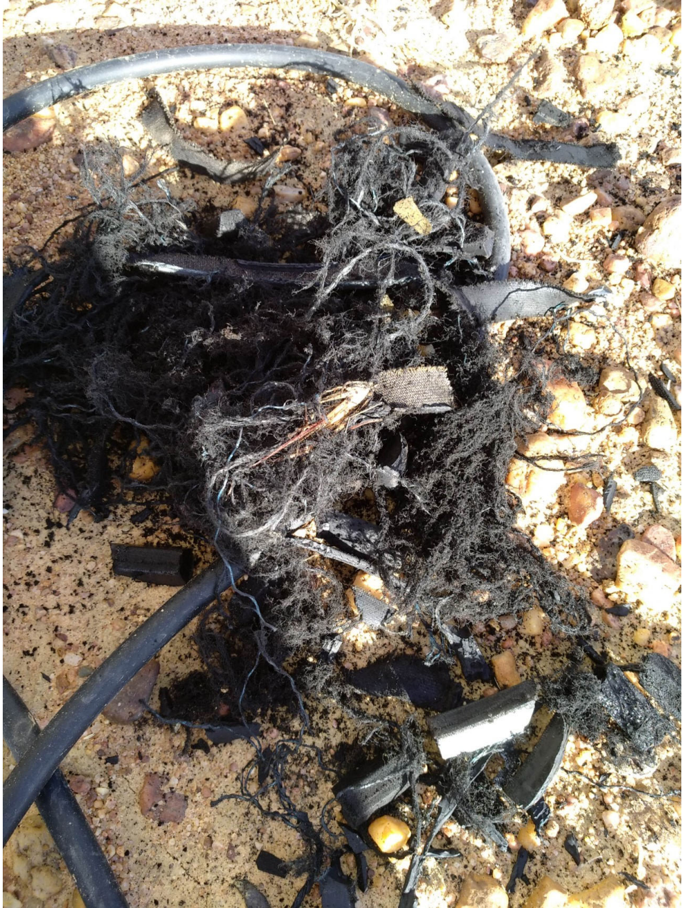
Figure 10: Wires damaged by cattle in the Ernest Henry South MIMDAS Survey.
