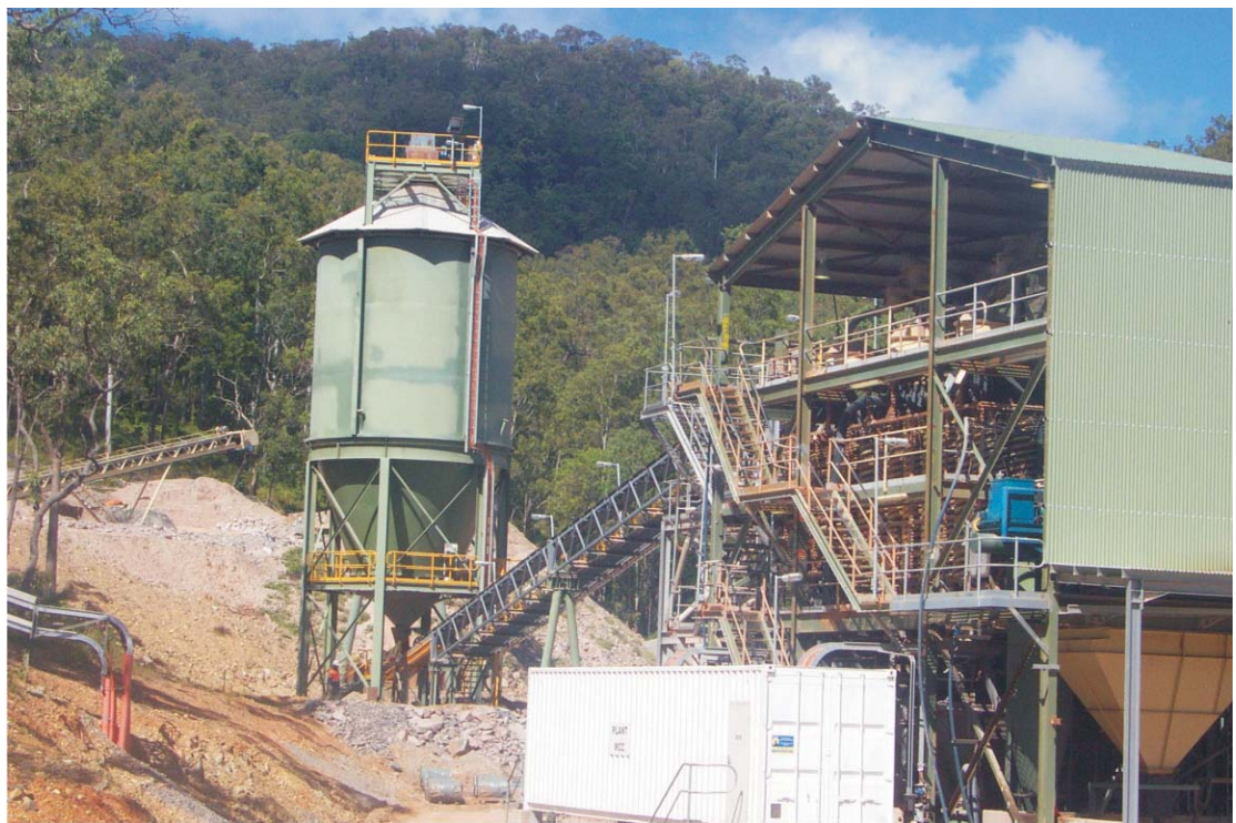
Plate 3: Collingwood treatment plant
