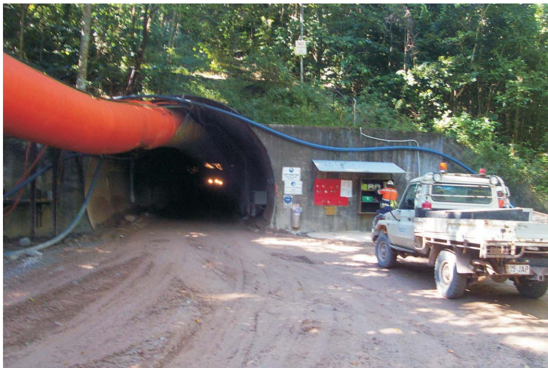
Plate 1: Collingwood adit portal
