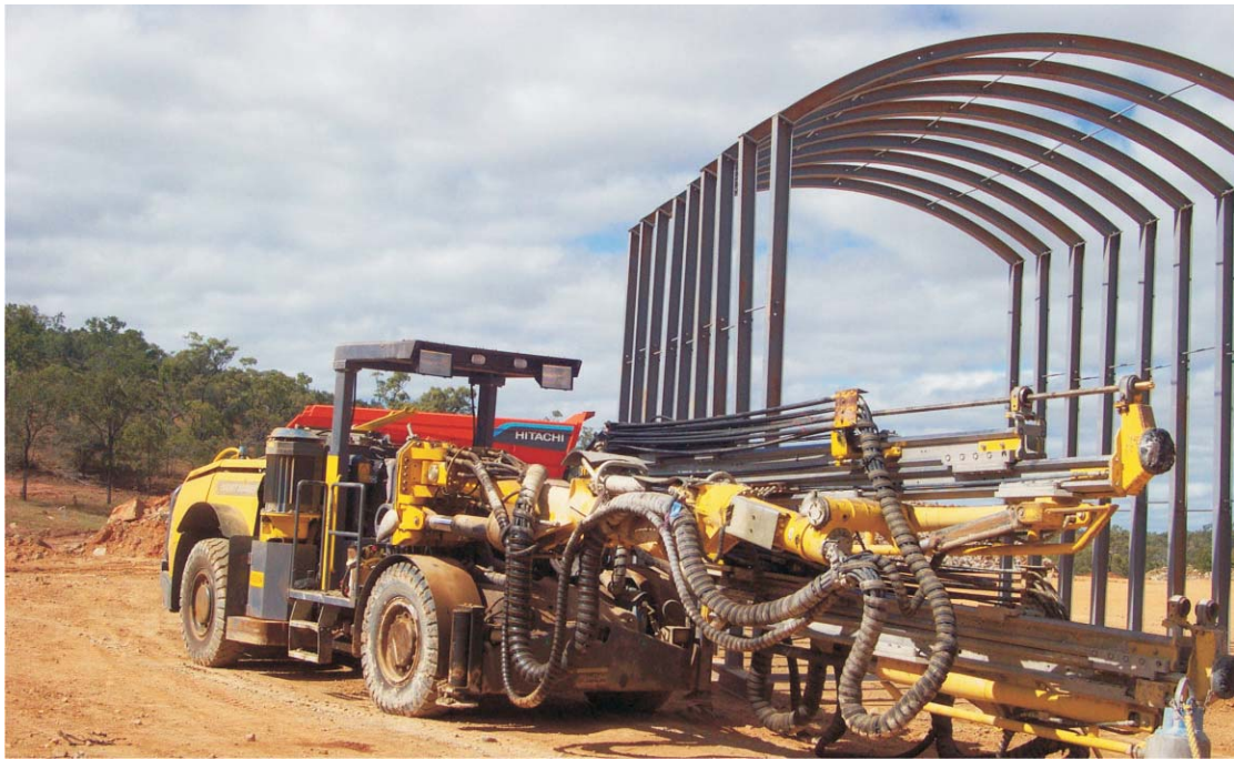
Plate 28: Mungana portal frame and machinery (photo taken 27/6/2006)
