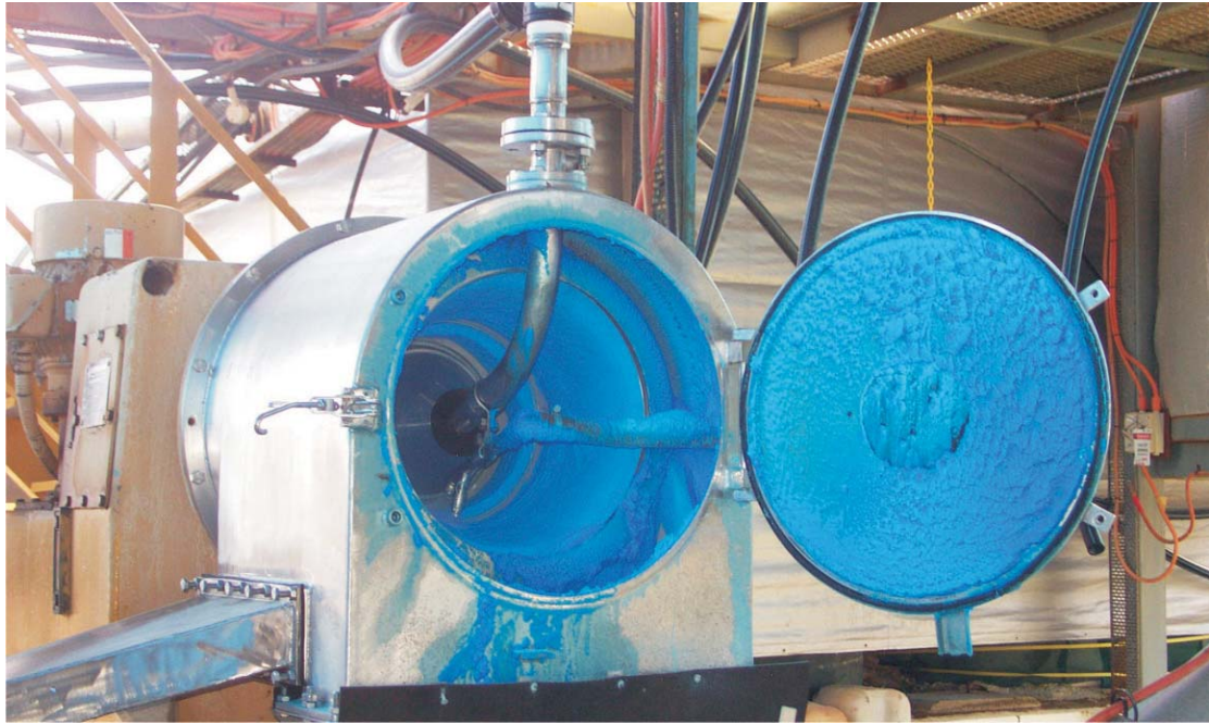
Plate 19: Tartana centrifuge copper sulphate (photo taken on 26/6/2006)
