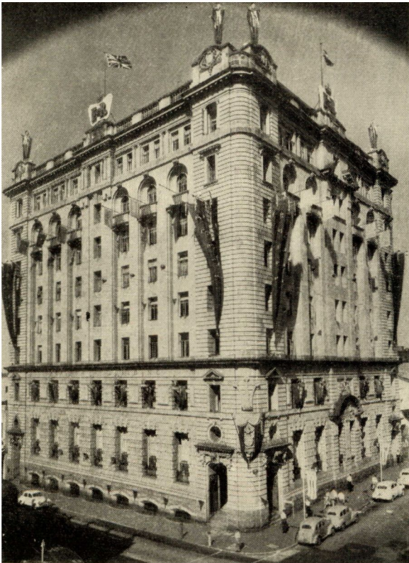
Taxation Building, George Street, Brisbane. —Base course of Greymare Granite, balance is Sandstone from Wright's Quarries, Helidon.
