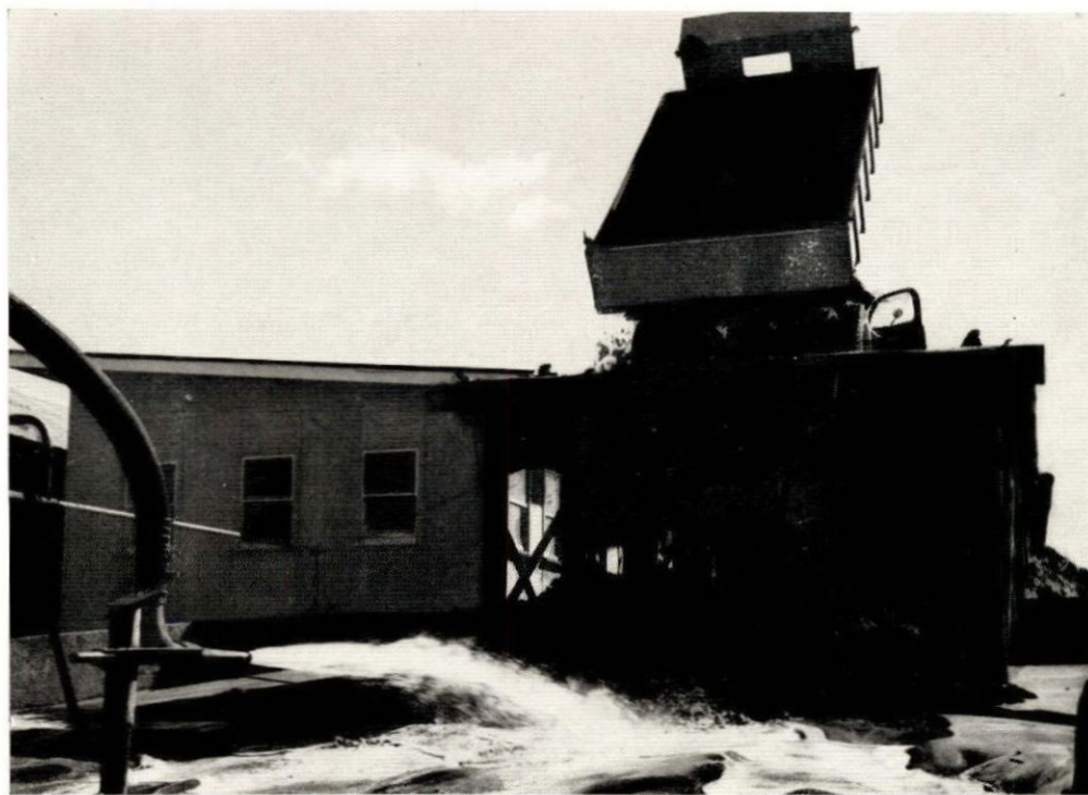
Plate 10, Fig. B Unloading Spiral Concentrate on to Ramp, whence it is pumped to Separation Mill, Mineral Deposits Pty. Ltd., Southport.
