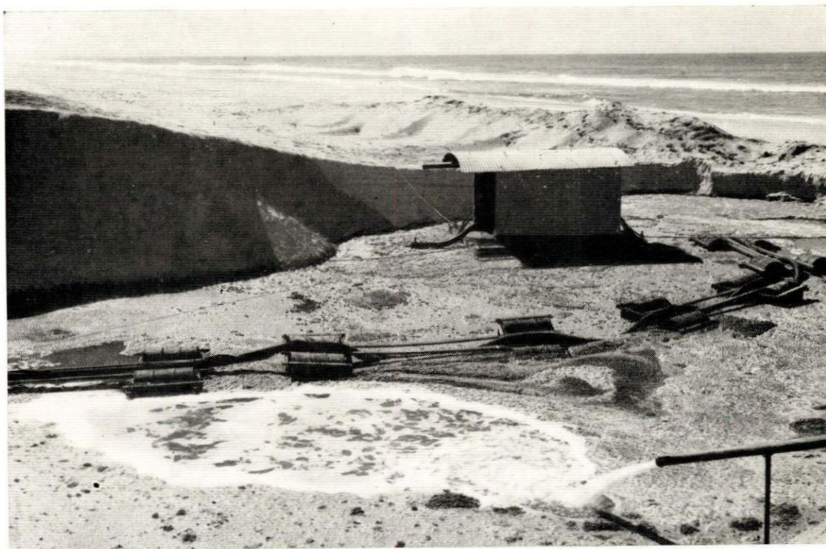
Plate 8, Fig. A Dredge Pond and Suction Dredge, Gold Coast.
