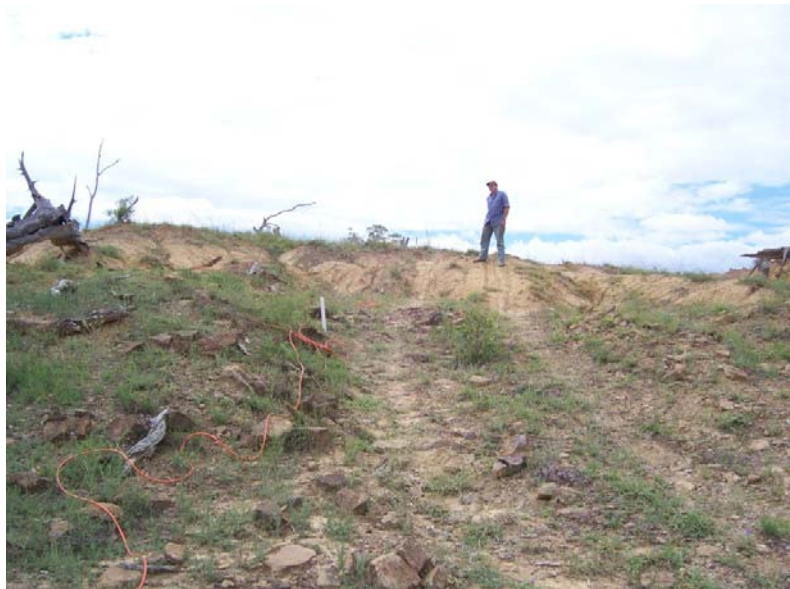
Vibe Tech checking steep bank for access
