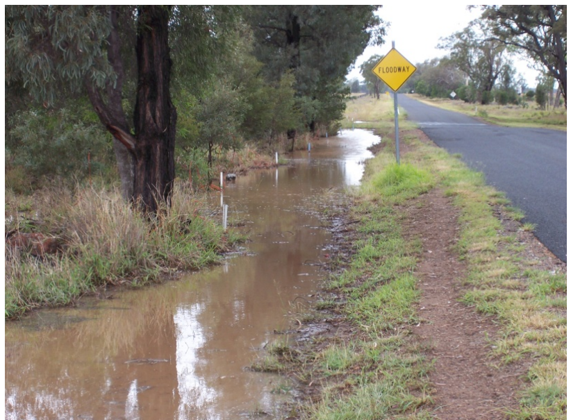
Water from recent rains lying alongside road
