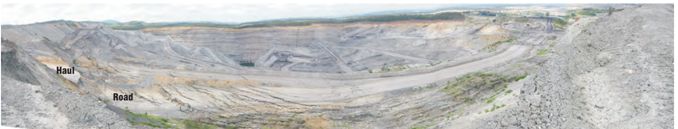
Figure 12: Mount Owen Low Wall failure (view from 215RL dump)
