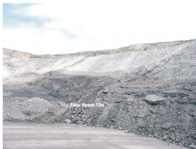
Figure 9: Mount Owen low wall post failure (in pit view)
