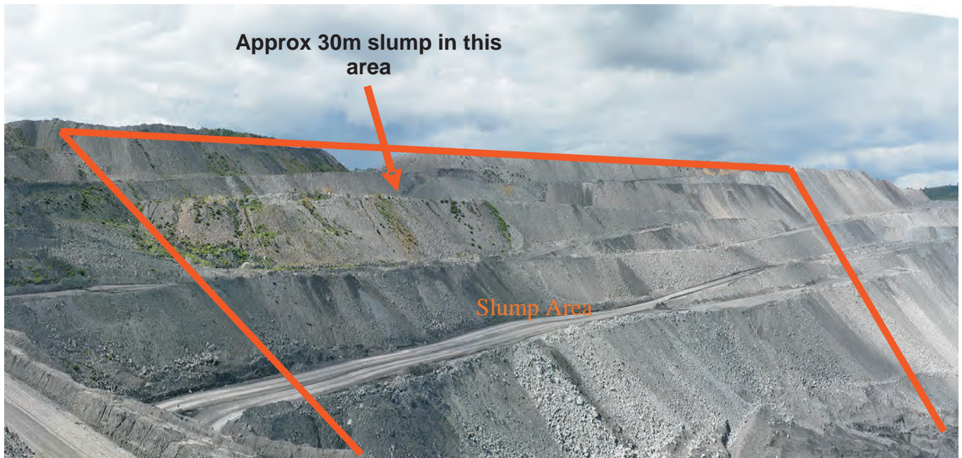
Figure 7: The slump area was approx 1km long and 200m high. The low wall slumped as a single entity causing a 30m slump at the top and a heave of 10–15m on the pit floor. Approximate mass of the slump was 30Mt.
