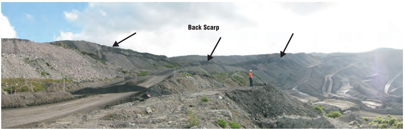
Figure 11: Mount Owen Low Wall Failure (view from B4 ramp)
