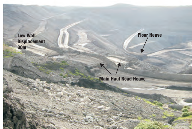
Figure 10: Mount Owen Low Wall Dump (Post Failure)
