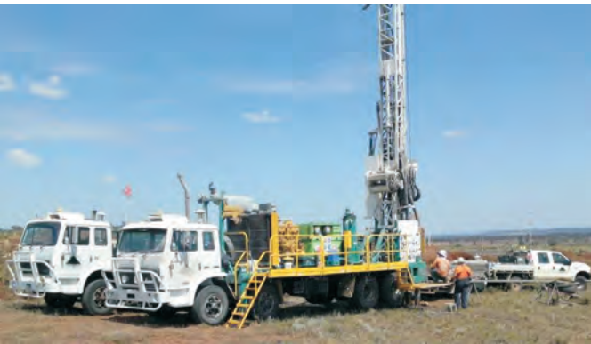
Figure 2b: Rig 2 after upgrade (May 2009)
