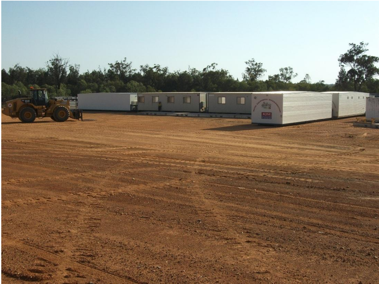
Picture 1: Camp under construction in Kurrajong Park, near Miles.
