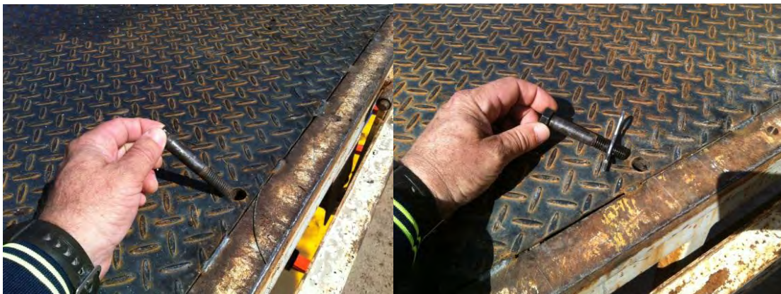
Figure 78. Ramp locking pin fitted to eliminate hazard
