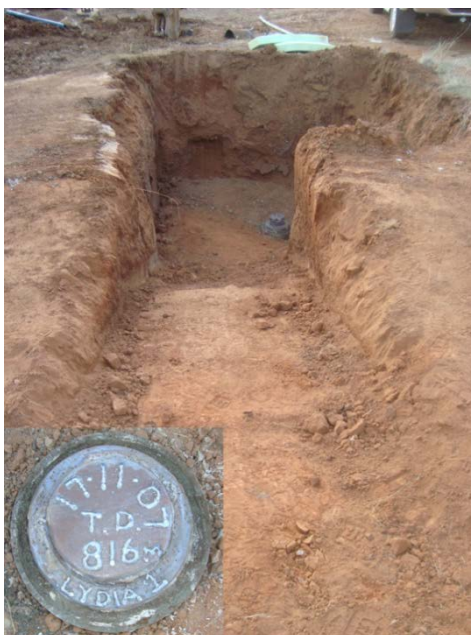
Figure 4 Lydia 1 Casing Sealed 1.5m below Ground
