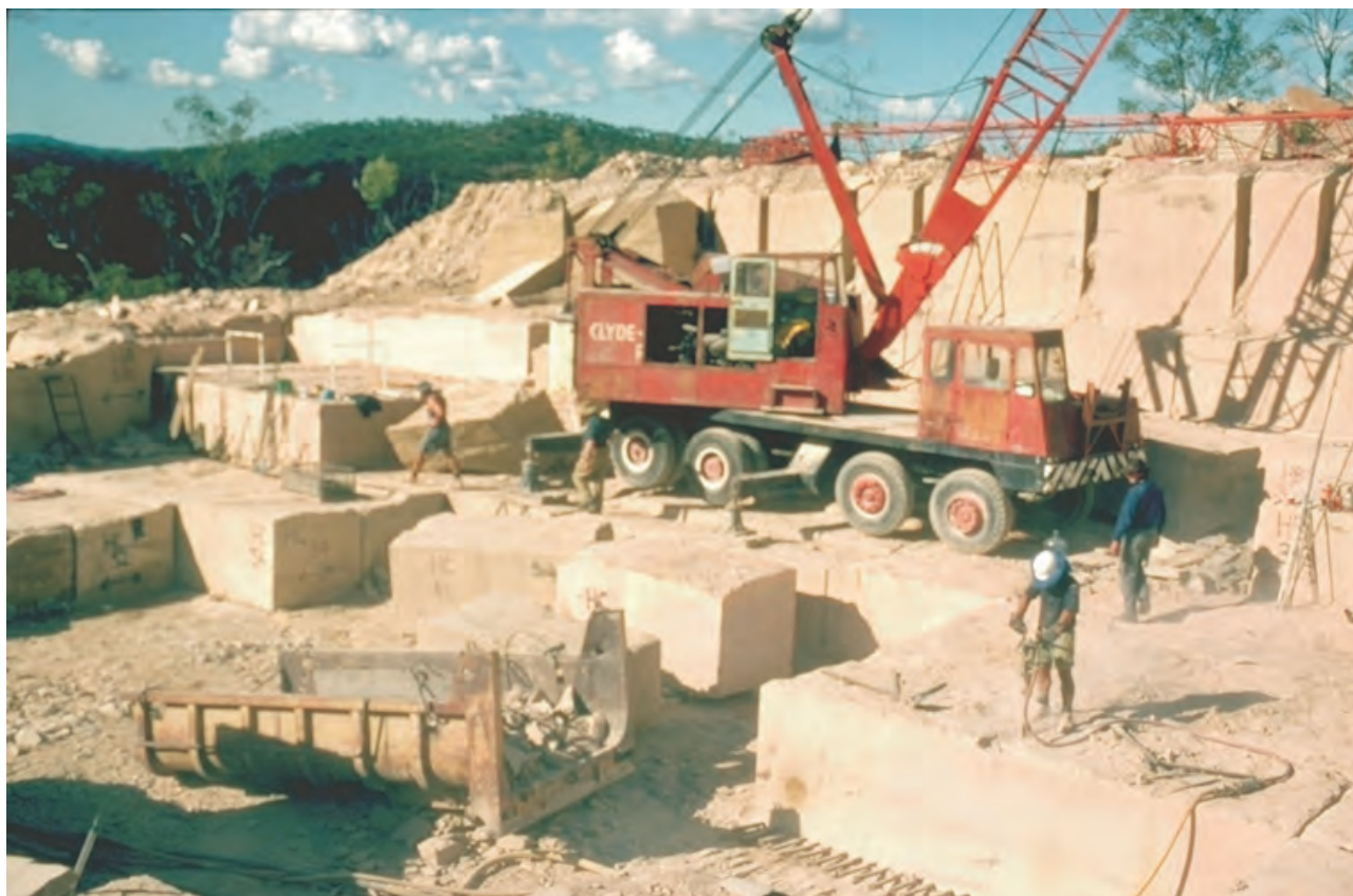
Figure 210. Sandstone quarry, Stanwell, 1997, Precipice Sandstone
