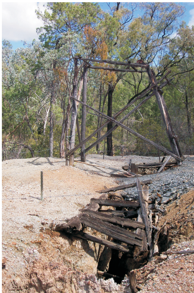
Figure 65. Headframe and shaft developed along Tooliambi lode
