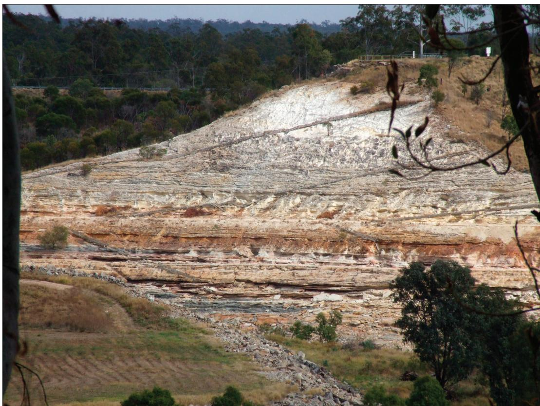
Figure 11. Spillway cut into the Freitag Formation at Fairbairn Dam
