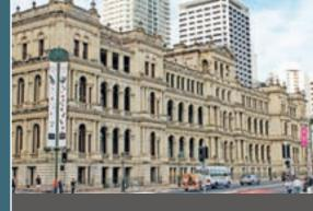
poor choice for a building stone: it is soft and therefore prone to weathering which has resulted in white colour that discolours easily and quickly appears dirty. The foundation is Brisbane Tuff from the O'Connelltown quarry, Fortitude Valley. The steps and floors of the Queen Street entrance, added in the 1950s are white marble (possibly from Rockhampton or New South Wales) and fossiliferous black marble (possibly from Windellama, New South Wales).
