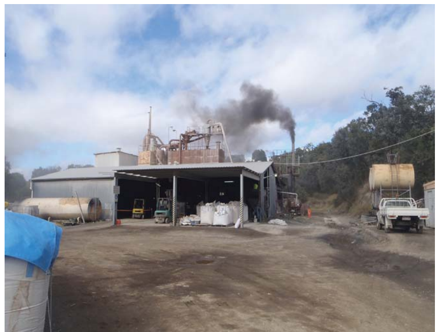
Photograph 187: Mount Sylvia bentonite processing and drying plant.
