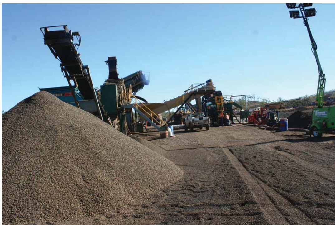
Photograph 138: Magnetite screening plant at Mount Moss.
