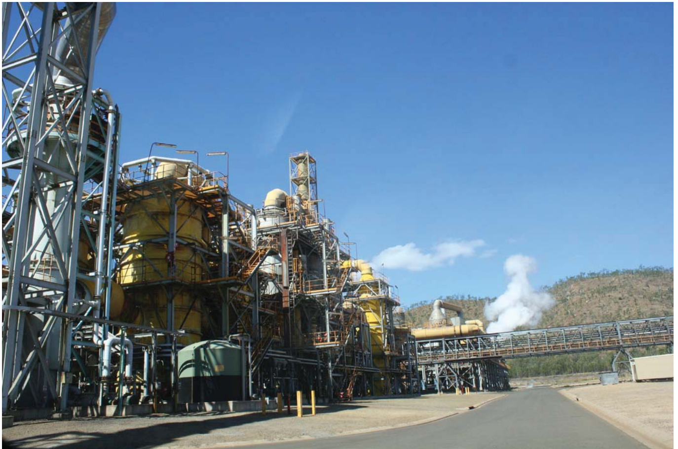
Photograph 13: Sun Metals Zinc Smelter – Townsville; roasting plant.
