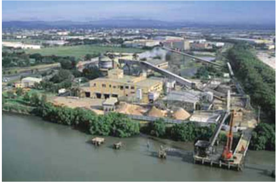
Photograph 223: Rutile, zircon and ilmenite products undergo final separation and clean-up at the dry mill at Pinkenba (image courtesy DNRM, Queensland Mineral and Petroleum Review, 2002).
