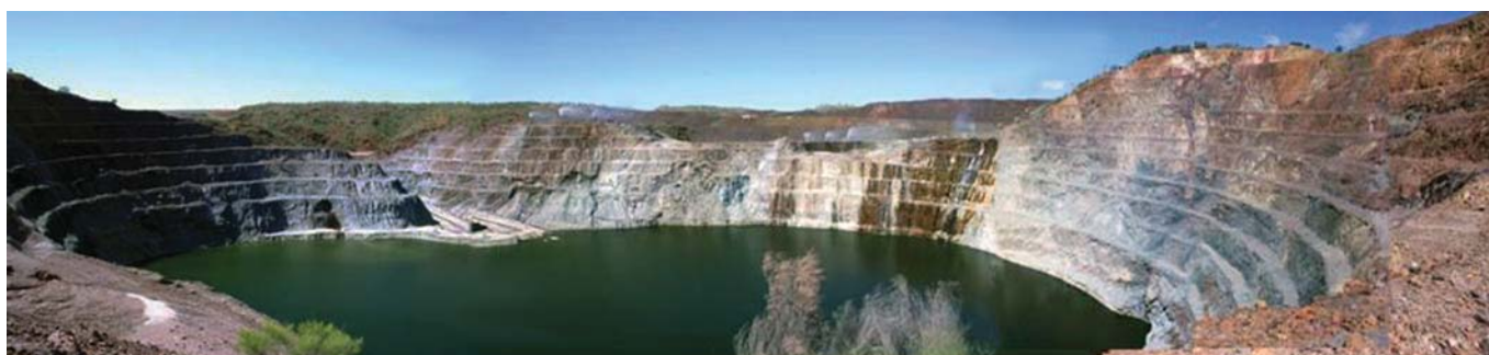
Photograph 25: The Esperanza open cut, currently used as mine water storage (panorama view).
