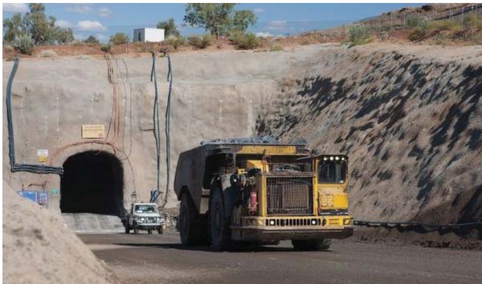
Photograph 80: Dugald River underground development portal (image courtesy of MMG Ltd).
