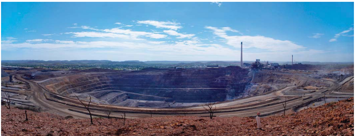
Photograph 72: Panorama view of the Black Star open cut with the Mount Isa mine infrastructure in the background (image courtesy DNRM).
