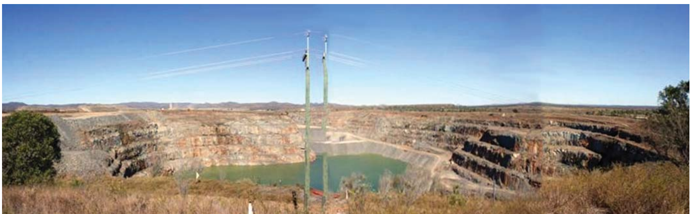
Photograph 107: Panorama view of the Sarsfield open cut in 2011, showing the plant in the background and waste refill in the back section of the pit.
