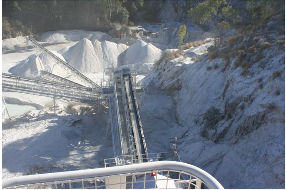
Photograph 200: Crushing operations at Bajool Marble mine.
