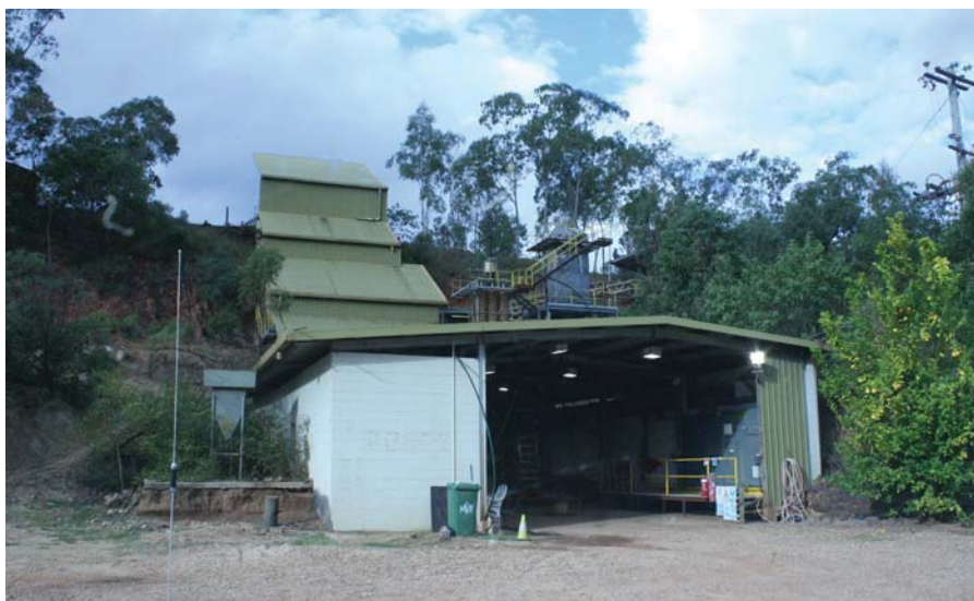
Photograph 151: General view of the Mount Veteran tin milling plant.
