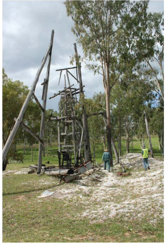
Photograph 144: Remains of the headframe and the mullock heap of the Wonbah Molybdenite mine, near Mount Perry.
