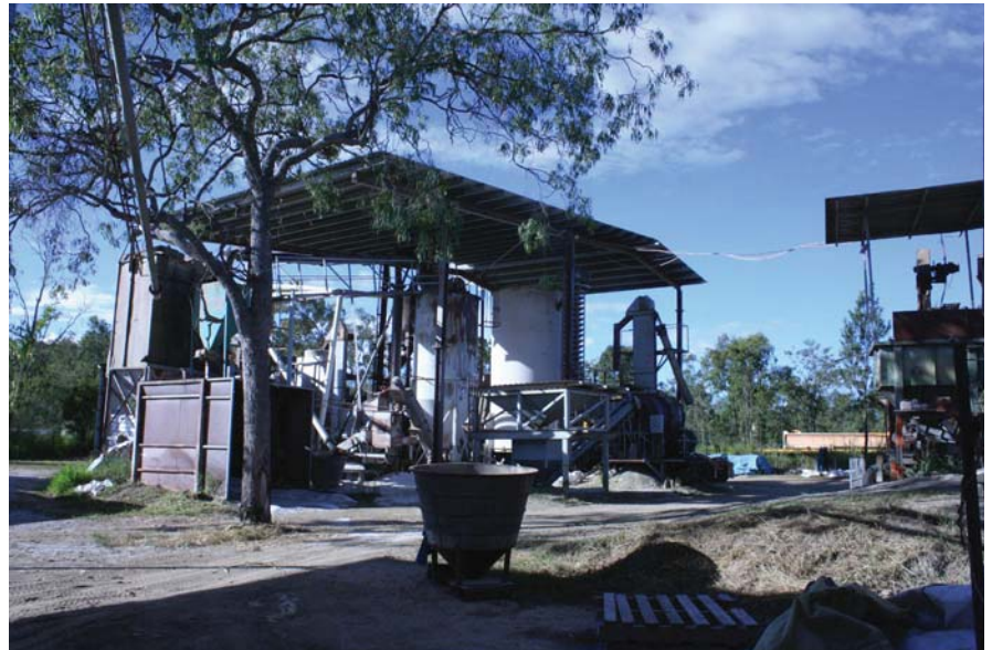
Photograph 210: The 'Chillagoe' perlite processing plant in Mareeba.
