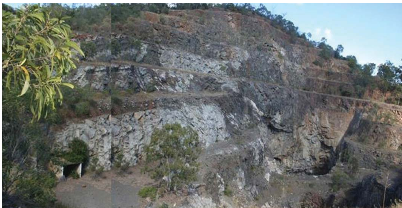
Photograph 140: Biggenden open cut and underground portal in 2009.
