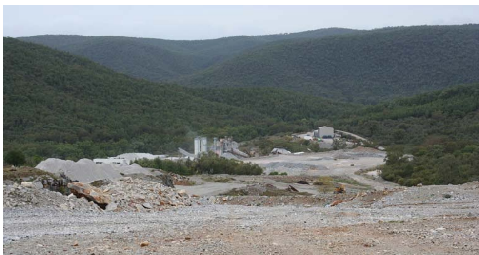
Photograph 194: Sibelco's Riverton limestone plant viewed from the limestone quarry.
