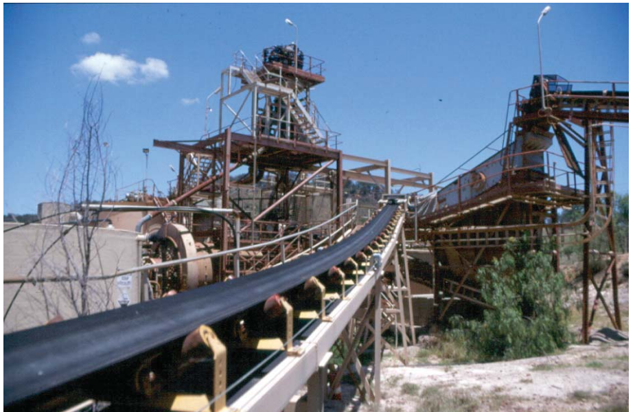
Photograph 124: Cracow Gold Mine plant in 'care and maintenance' in 1997, as operated by the Cracow Mining Venture.
