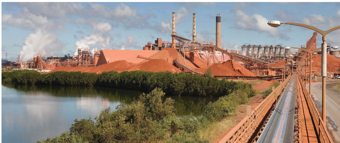
Photograph 9: Queensland Alumina Refinery — Gladstone (© Bruce Peebles 2008).
