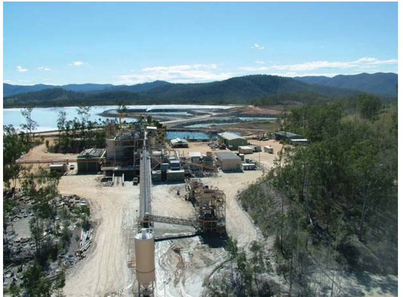
Photograph 111: Treatment plant at Mount Rawdon (image courtesy David Carmichael, DNRM).
