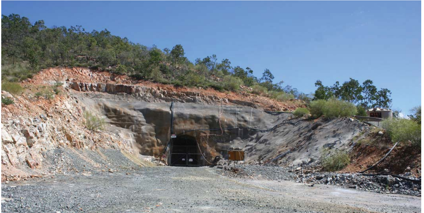
Photograph 87: The West 45 underground portal.
