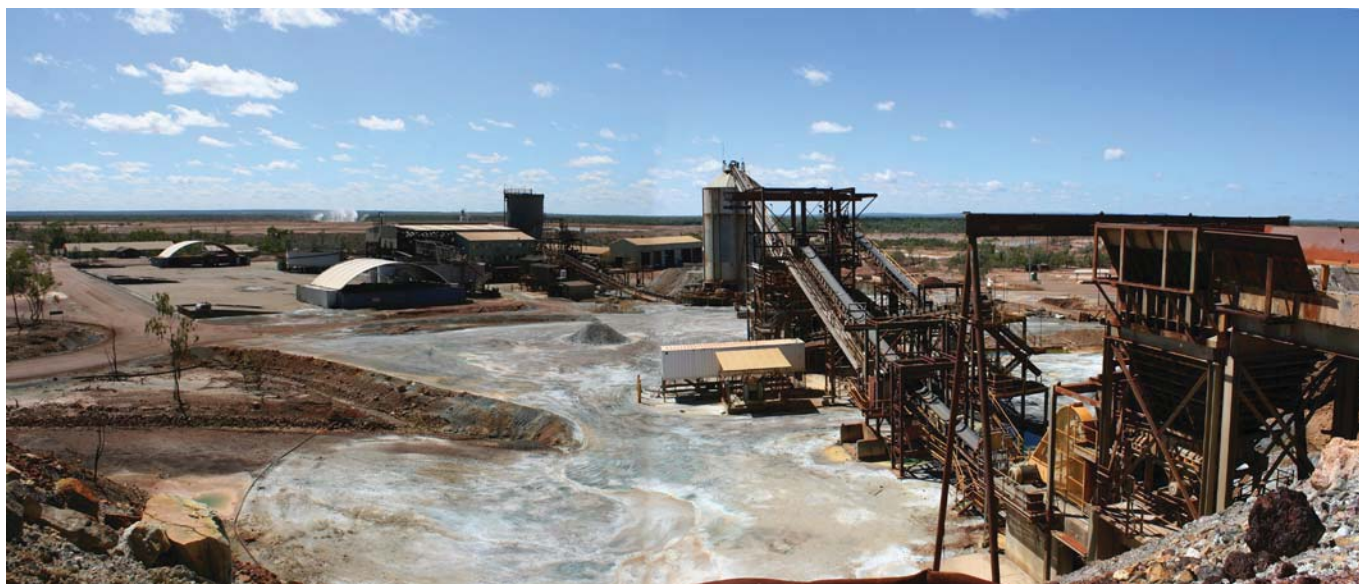
Photograph 85: Thalanga processing plant viewed from the ROM pad near the primary crusher.
