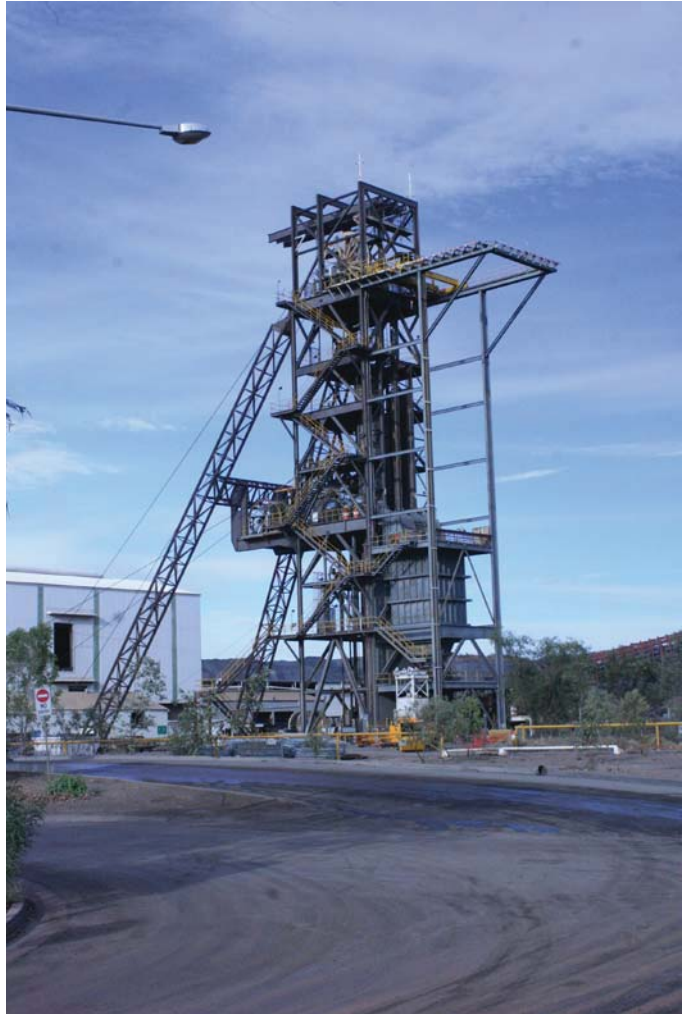
Photograph 74: Headframe of George Fischer Mine.
