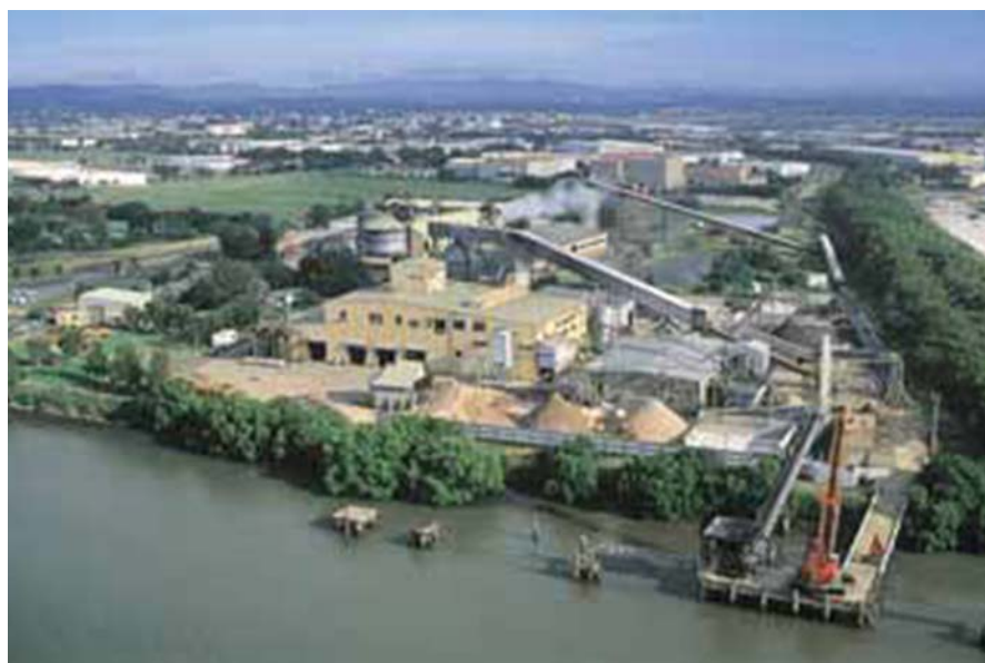
Photograph 287: Rutile, zircon and ilmenite products undergo final separation and clean-up at the dry mill at Pinkenba (image courtesy DNRM, Queensland Mineral and Petroleum Review, 2002).
