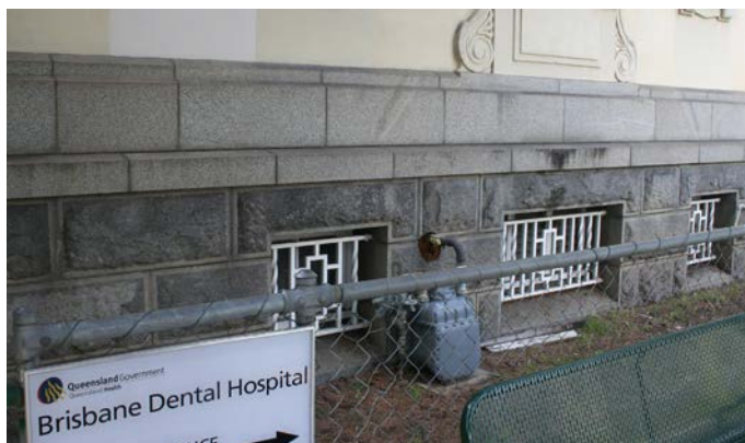
Photograph 233: (a) A bluish-grey, mafic biotite hornblende quartz diorite, which darkens on polishing, associated with the Bouldercombe Igneous Complex. This dimension stone clads the base course of the Dental Hospital in Turbot Street in Brisbane and was sourced from Gracemere quarry near Rockhampton. (b) The Dental Hospital on Turbot Street.
