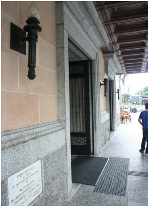
Photograph 232: (a) Granite base course and granite railings at the main façade of the Old City Hall, Brisbane, comprising equigranular biotite granodiorite with distinctive mafic enclaves associated with the Samford Granodiorite from the Camp Mountain deposit, near Mount Nebo, north of Brisbane; (b) Main entrance of the Old City Hall, Brisbane, clad with Samford Granodiorite from Camp Mountain.
