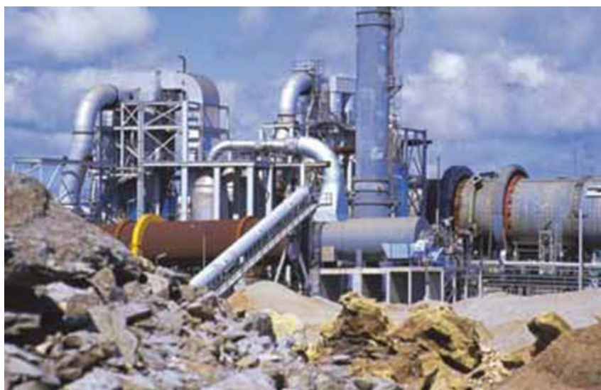
Photograph 298: Stage one Stuart Oil Shale plant; rotary dryer and processor (image courtesy QER Pty Limited, Queensland Mineral and Petroleum Review, 2002)
