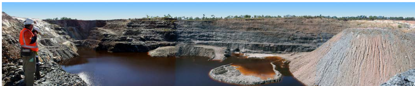
Photograph 58: Panorama view of the Surveyor open cut with underground portal and waste dump refill on right of view.
