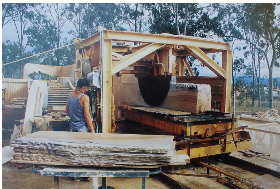
Photograph 218: 1988 Diamond-bladed block saw. Lockyer Sandstone Pty Limited (image courtesy David Trezise).
