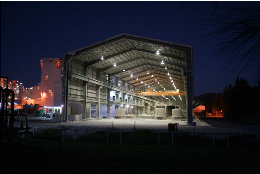
Photograph 268: Parkhurst magnesia processing plant near Rockhampton.
