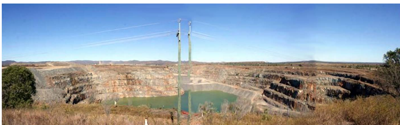
Photograph 117: Panorama view of the Sarsfield open cut in 2011, showing the plant in the background and waste refill in the back section of the pit.
