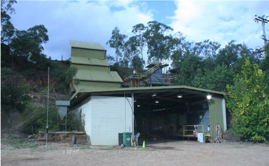
Photograph 173: General view of the Mount Veteran tin milling plant.
