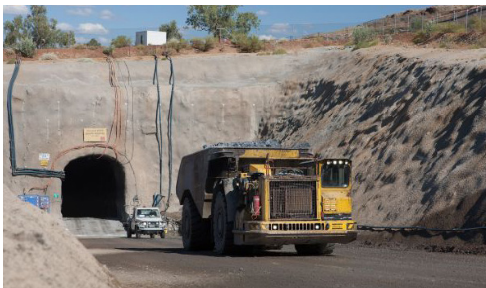
Photograph 80: Dugald River underground development portal (image courtesy of MMG Ltd).
