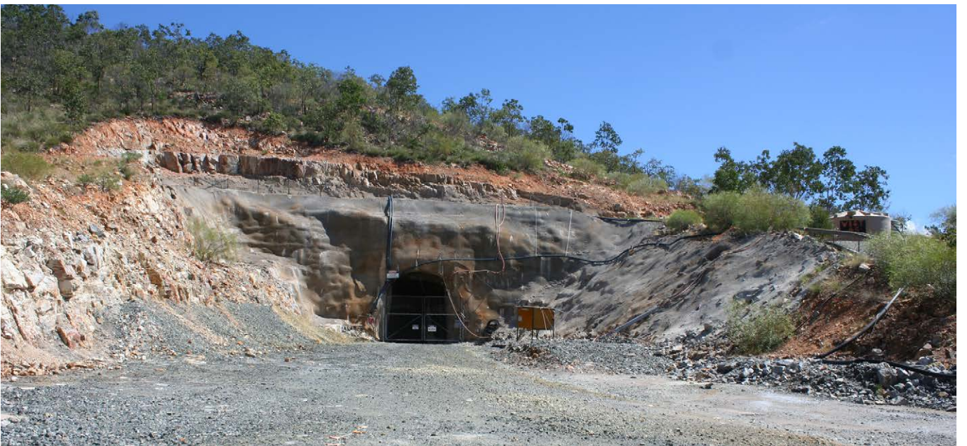
Photograph 88: The West 45 underground portal.
