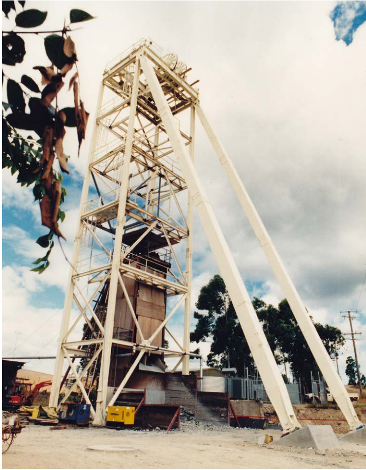
Photograph 120: Headframe of the Gympie Scottish Nr.2, around 1996.
