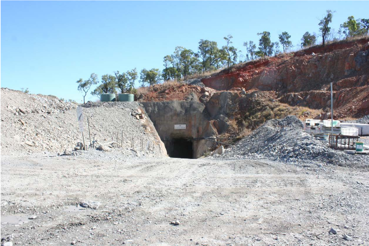
Photograph 93: Portal of Mungana underground zinc mine.
