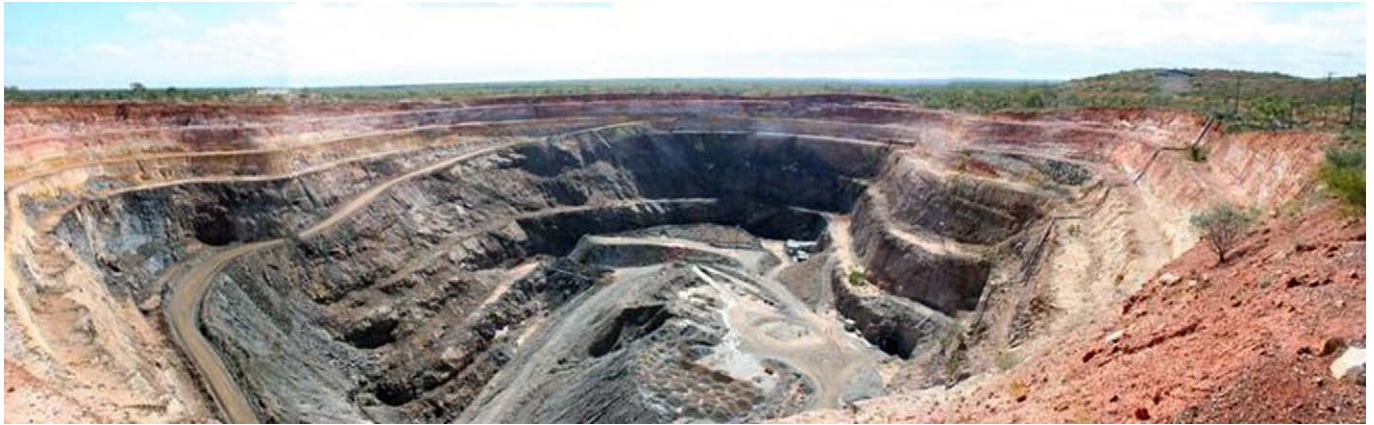
Photograph 37: Osborne open cut with underground portal at the base of the pit.
