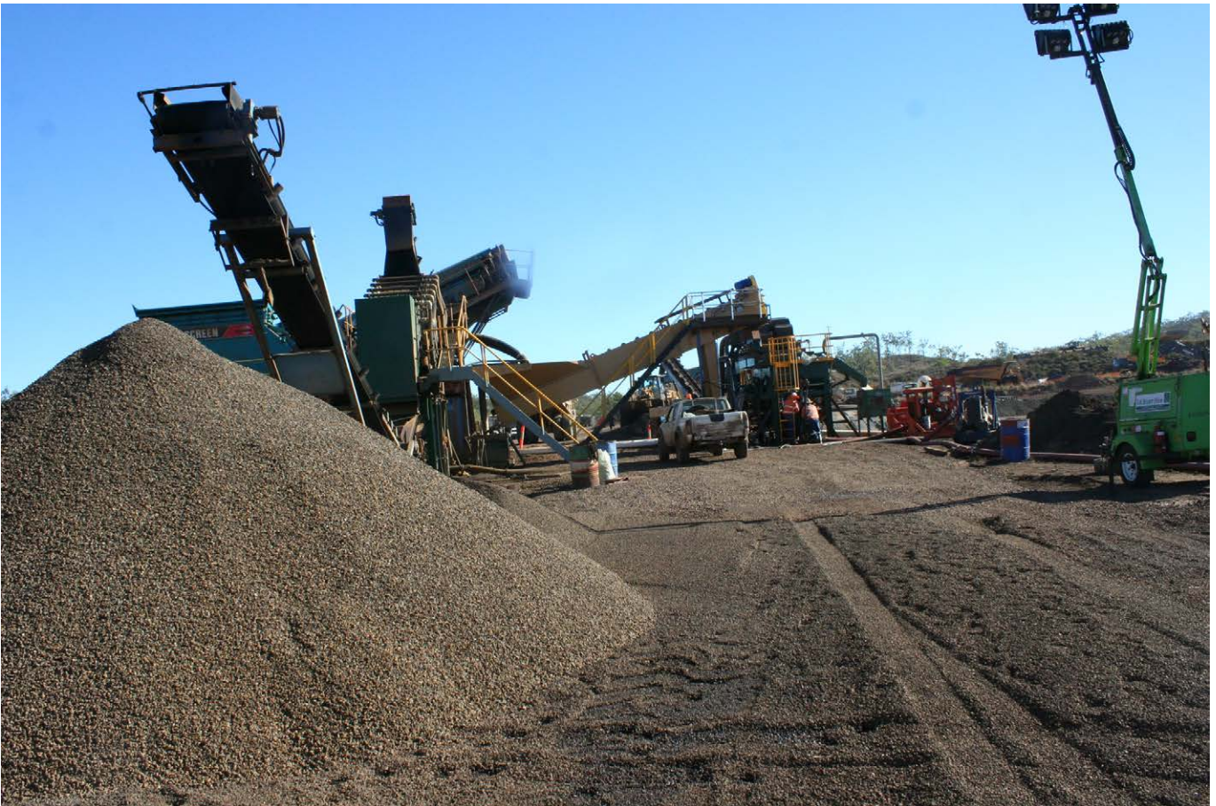
Photograph 152: Magnetite screening plant at Mount Moss.
