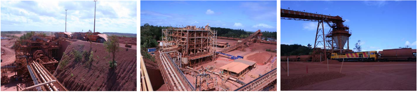
Photograph 20: Andoom bauxite processing plant, (left) dump bridge hopper feeding bauxite into a scrubber and trammel; (centre) Andoom fines separation plant; (right) product conveyor and load out bin for train transport to Port of Weipa.
