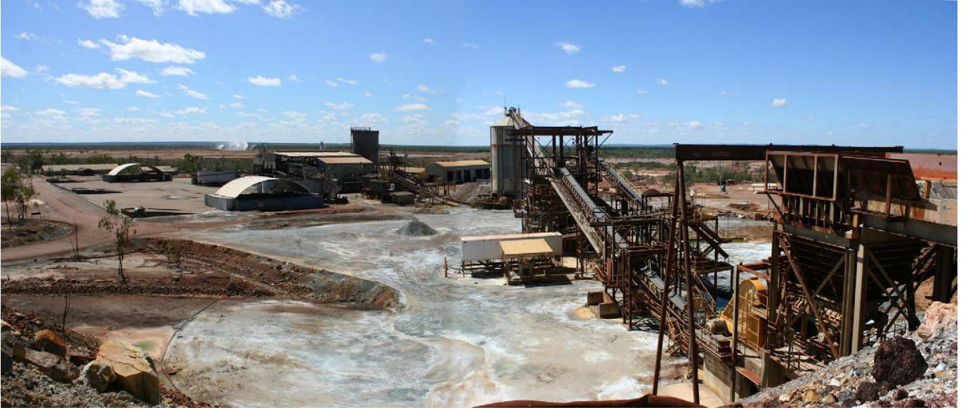
Photograph 86: Thalanga processing plant viewed from the ROM pad near the primary crusher.
