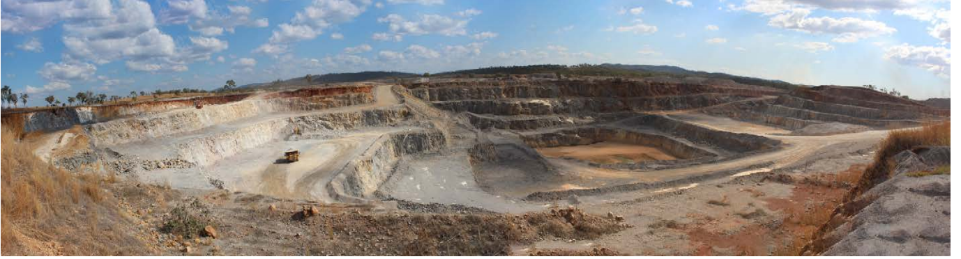
Photograph 260: Taragoola open cut within highly fractured grey limestone.
