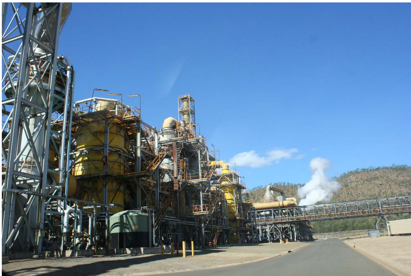
Photograph 13: Sun Metals Zinc Smelter – Townsville; roasting plant.
