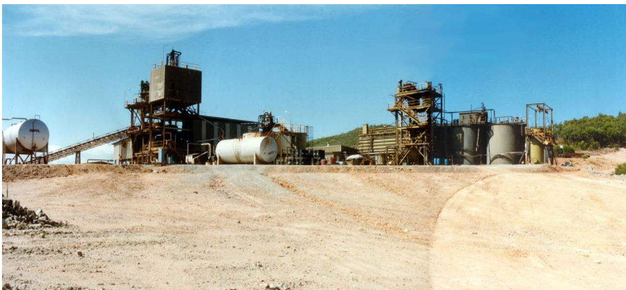
Photograph 128: Horn Island Gold Mine plant in 1990.
