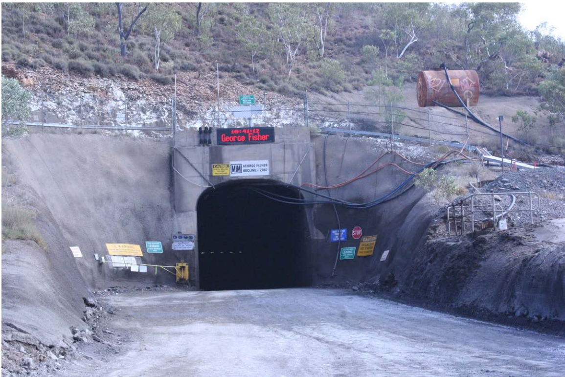
Photograph 75: Underground entry to the George Fischer Mine with access to the North and South deposits.
