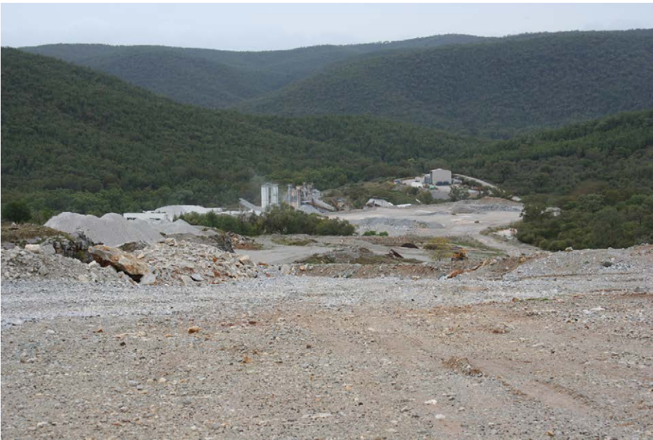
Photograph 261: Sibelco's Riverton limestone plant viewed from the limestone quarry.
