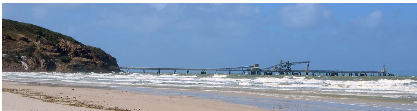
Photograph 7: Port of Cape Flattery (image courtesy Bob Bultitude, GSQ).
