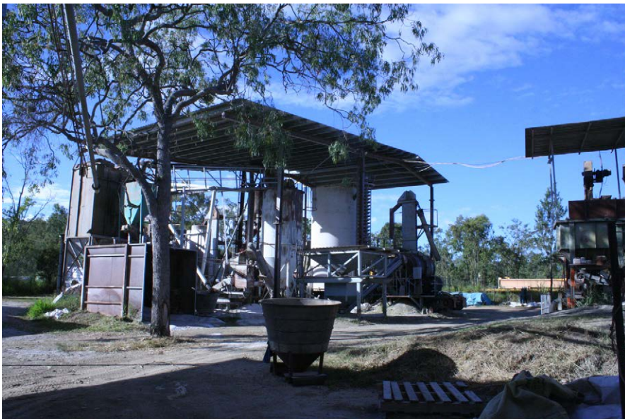
Photograph 274: The 'Chillagoe' perlite processing plant in Mareeba.
