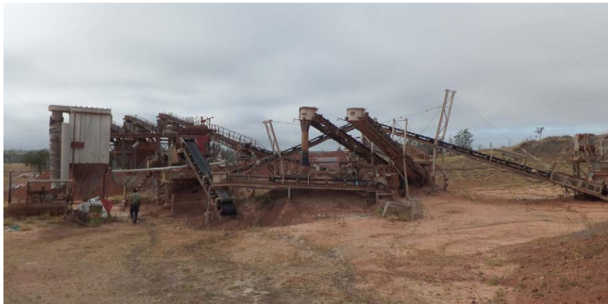
Photograph 293: Queensland Zeolite's processing plant at Willow zeolite mine.
