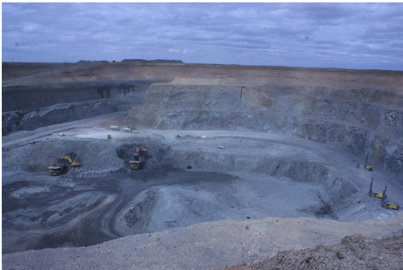
Photograph 47: The E1 open cut at Mount Margaret.
