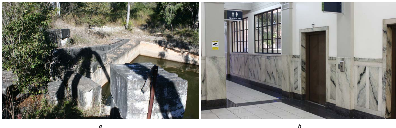
Photograph 223: (a) Historic marble pit at Ulam adjacent to current Bajool Marble east pit, which is considered the source location for marble cladding used in prominent Government buildings in Brisbane – see also Photograph 258; (b) Cladding of internal hallway within the State Government building along Adelaide Street in Brisbane comprise of the greenish-black and white streaked Ulam marble.
