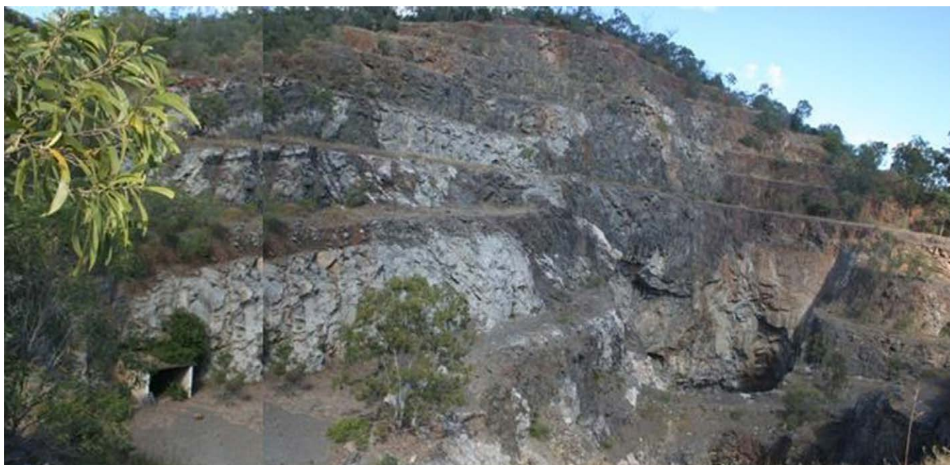
Photograph 154: Biggenden open cut and underground portal in 2009.
