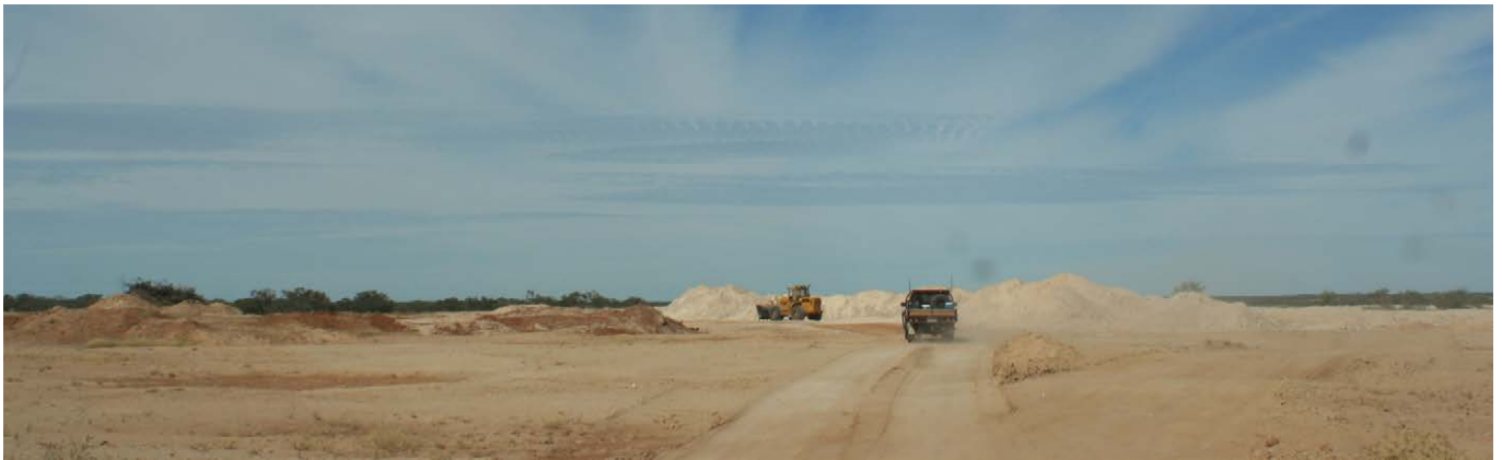
Photograph 254: Surface excavations at one of the Cork gypsum deposits held by Zinaback Pty Limited in the Winton district.
